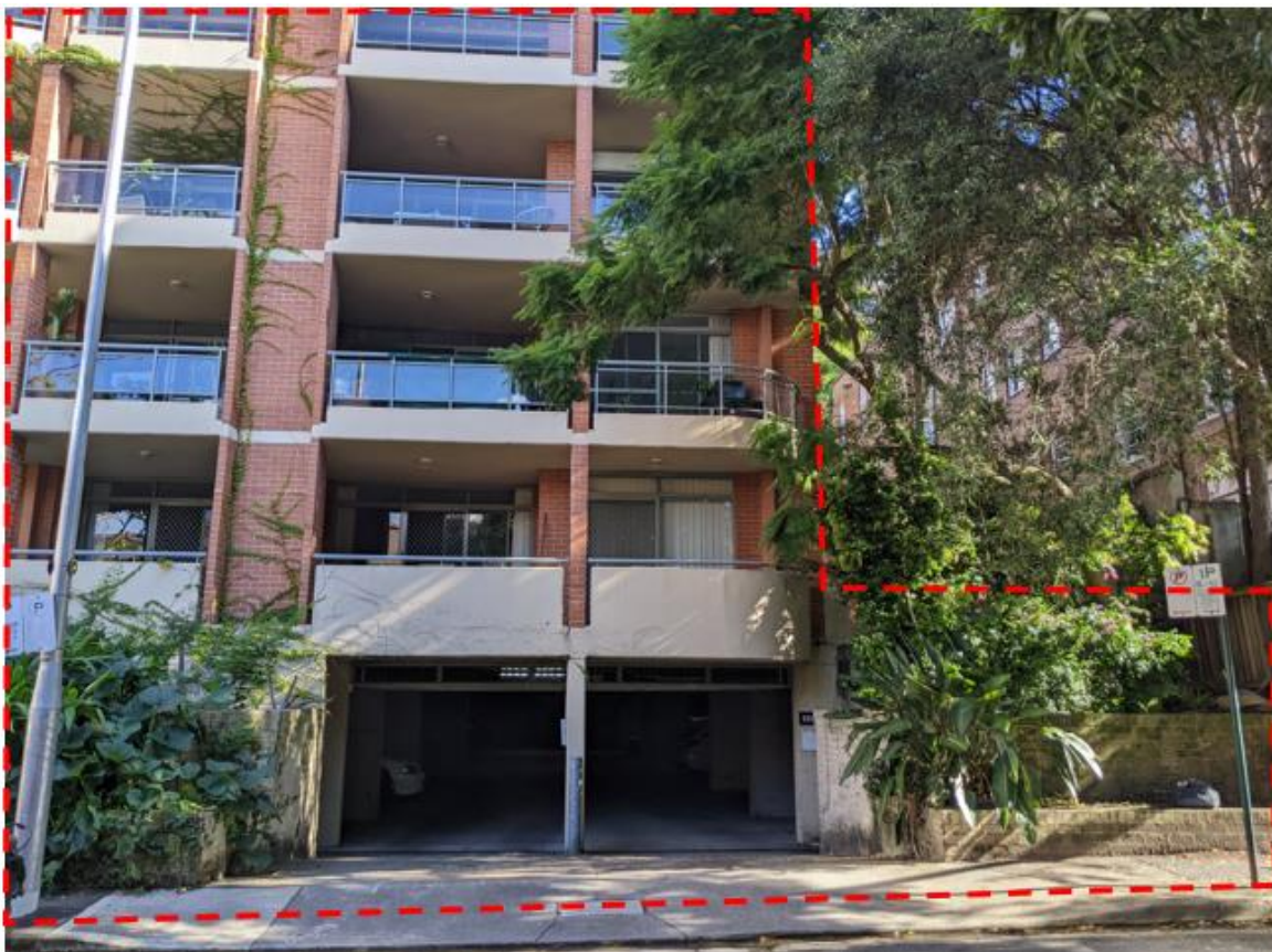
Figure 4: Existing double crossover vehicle access to basement from Billyard Avenue
