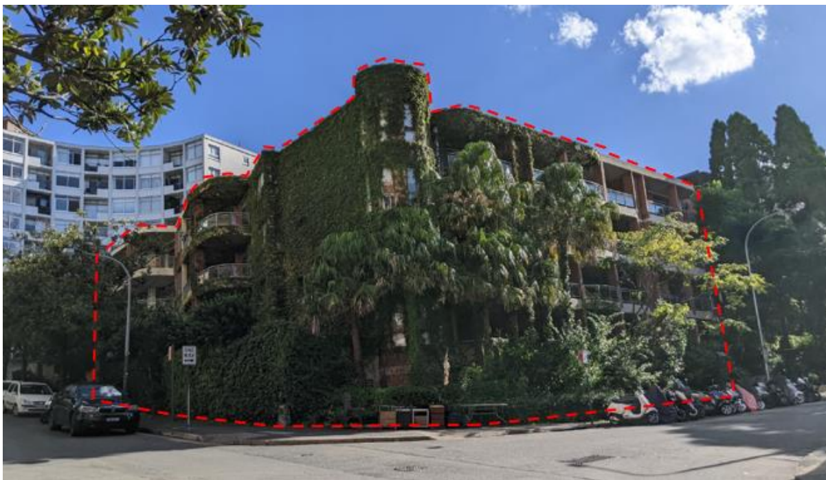
Figure 2: Subject site viewed from the intersection of Lithaca Road and Billyard Avenue
