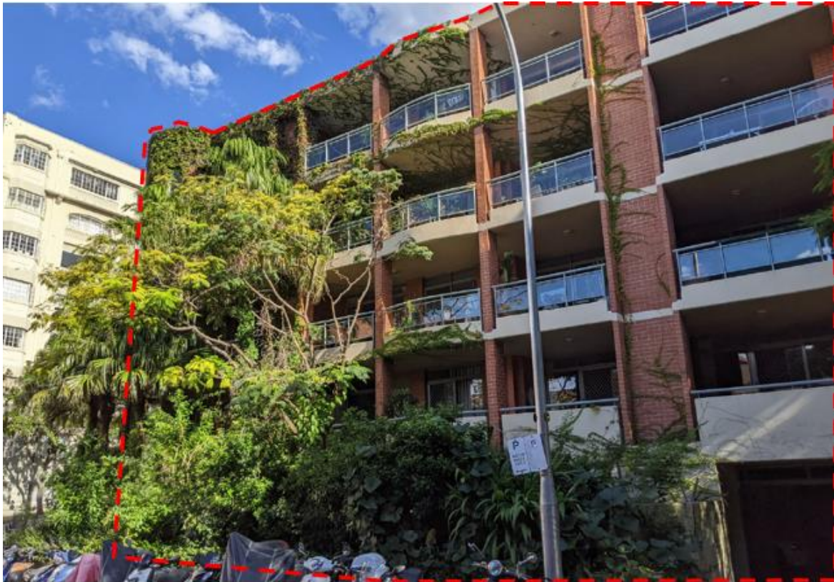
Figure 3: Front (north) elevation of site viewed from Billyard Avenue
