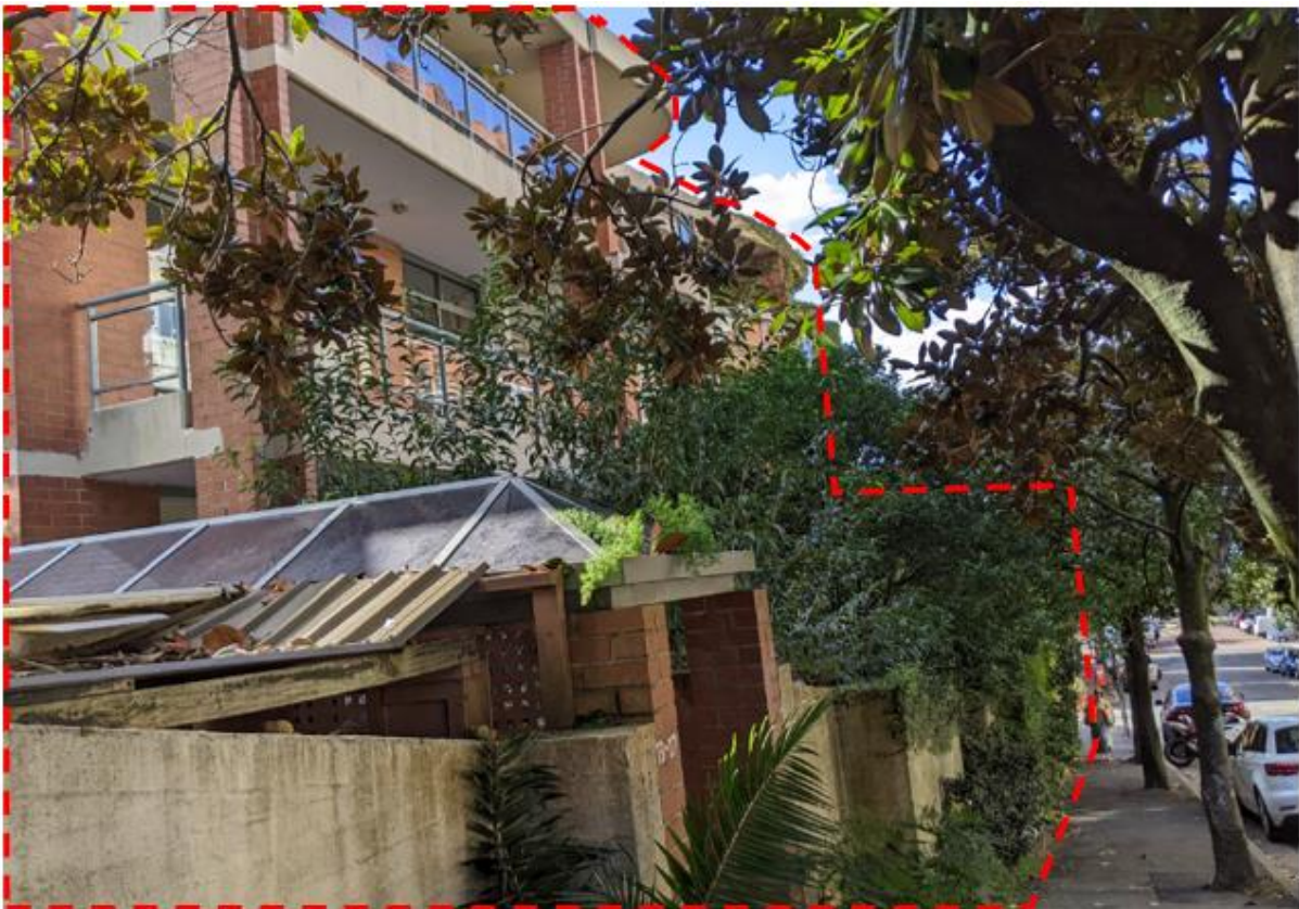
Figure 6: Existing pedestrian entry from Ithaca Road
