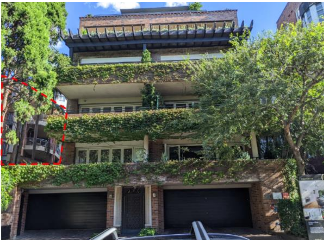
Figure 8: Front of No.27 Billyard Avenue, adjacent neighbour to the west of the subject site
